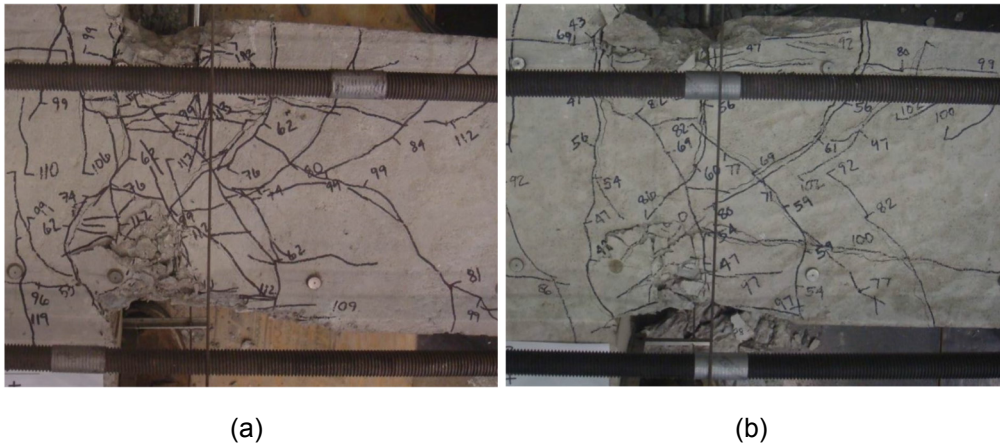
Figure 4-8 Column specimens at first excursion to drift ratio of 4% (Rautenberg, 2011): (a) Specimen CC-3.3-20, with Grade 60 reinforcement; and (b) Specimen UC-1.6-20, with Grade 120 reinforcement.
